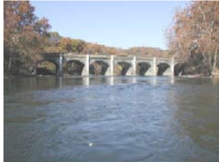
“Rail bridge near Ryde, PA on the Juniata River” (Clark Fisher)
