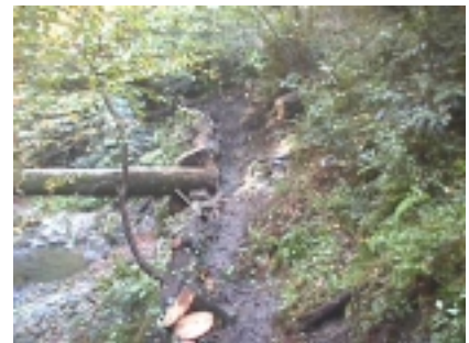
Work completed, original trail route open
